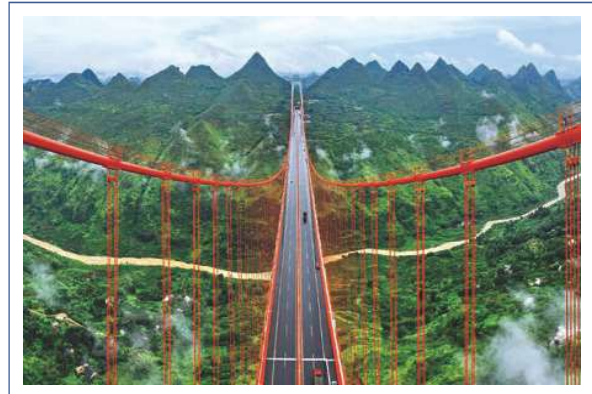
坝陵河大桥 Baling River Birdge
